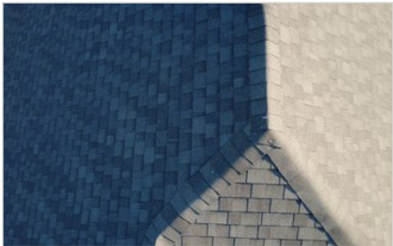
Three-plane hip junction with cap shingles.
